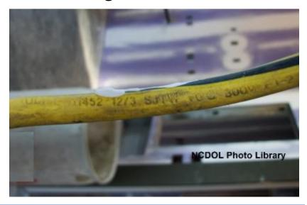
Conductors entering boxes, cabinets, or fittings must be protected from abrasion
